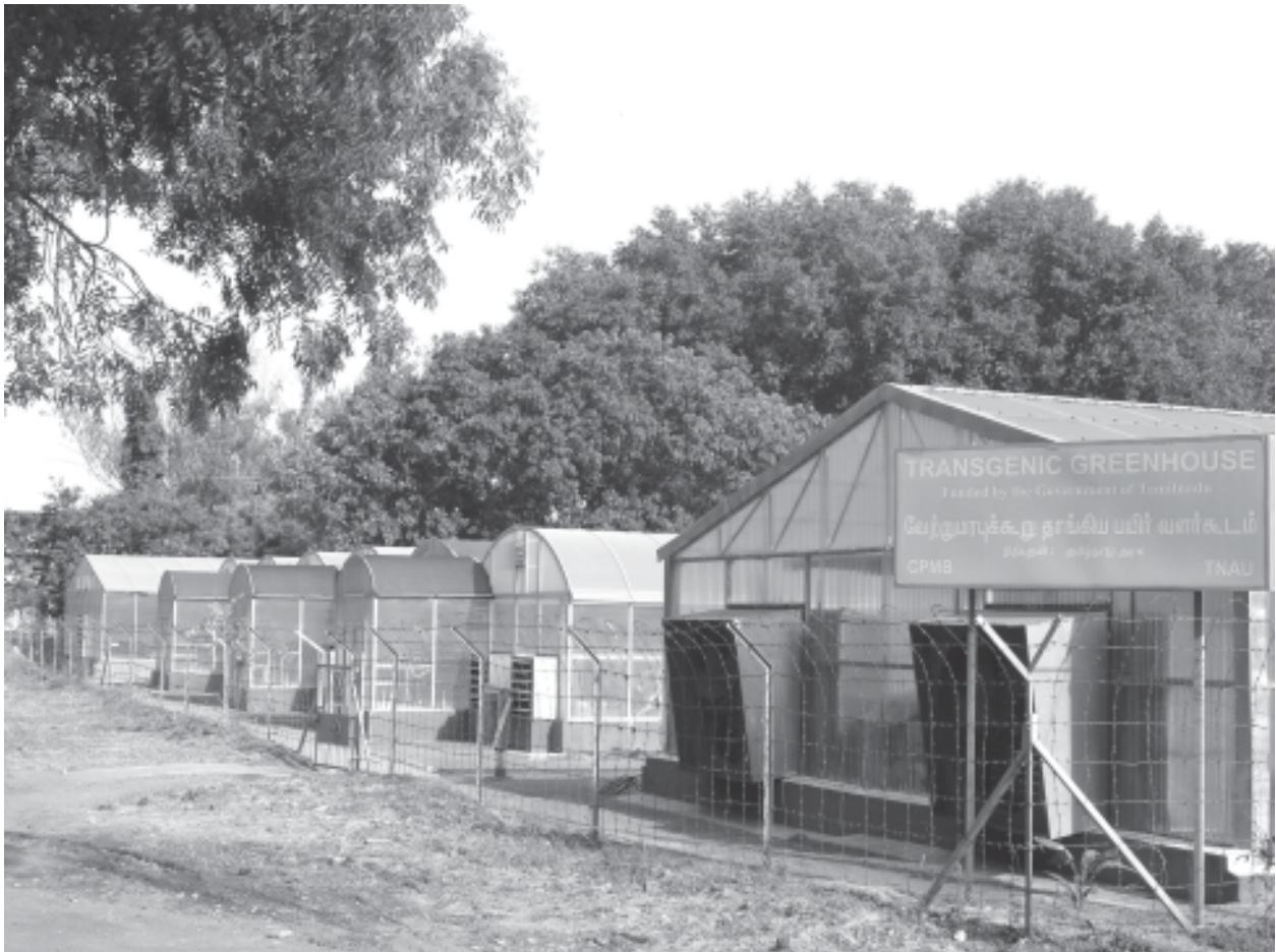
Figure 20. Transgenic greenhouse facilities at TNAU, Coimbatore
